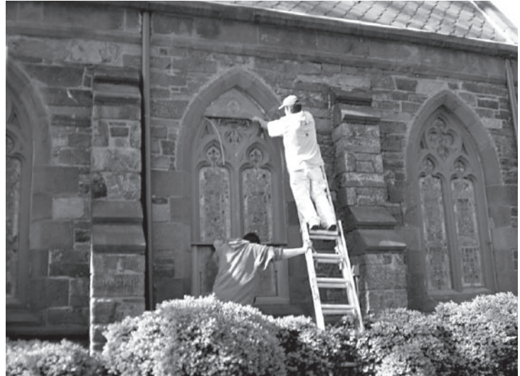
Workmen remove lexan panels covering the Renwick Chapel windows.
