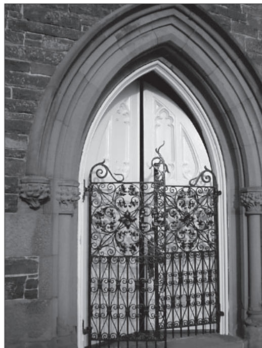
Main doors and gates of the newly refurbished Renwick Chapel.
