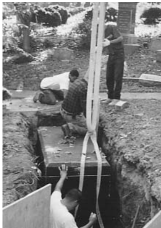
New Pathway Crypts being installed.
